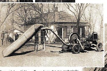
Dust settled so thickly on Kansas lawns that two mechanicallyinclined men started a profitable business with the huge homemade outdoor vacuum cleaner shown above. Right—Typical scene along silt-covered road in the sand-swept Great Plains area.
