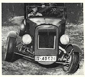
Swaying or tilting when driving around curves or over bumpy roads is claimed to be eliminated with this "curve-balancer." Metal elbows allow independent movement of the wheels.
