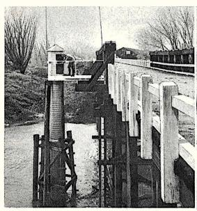
Photo above shows semi-portable gauge in Californian stream. Right—I. M. Ingerson is seen with transmitter and keying device which broadcasts warnings when water level increases.
