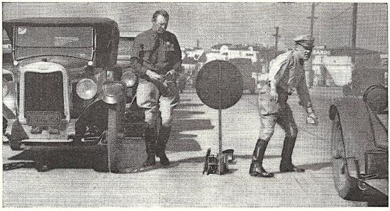
Seeking killer cars, California Highway Patrol officers stop all autos suspected to be in bad condition, and immediately test brakes. A brake testing box is clamped to the running board, the car is speeded up, and then stopped suddenly at the officer's command. Impact of sudden stop swings pendulum inside box, meter showing stopping distance from 20 m.p.h. speed.
