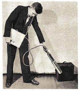
The old electroscope method of locating lost radium is being replaced by the portable outfit above. Instrument needle in box is deflected when the rod finds the precious metal.
