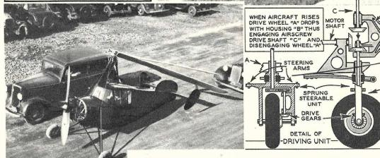
Drive wheel A in above diagram would propel flying automobile on land. To take off giro blades are started spinning and drive wheel runs the car for short distance needed for autogiro takeoff. In flight, wheel would drop, engaging shaft C which drives propeller for forward flight. Photos show latest wingless Pitcairn autogiro. The government has ordered similar ships with geared wheels.
