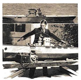
Top—Model of S. S. Saratoga. Photoelectric cell in smoke stack controls boat in calm water. Lower photo shows relative size of copper plated ship which took 300 hours to build.
